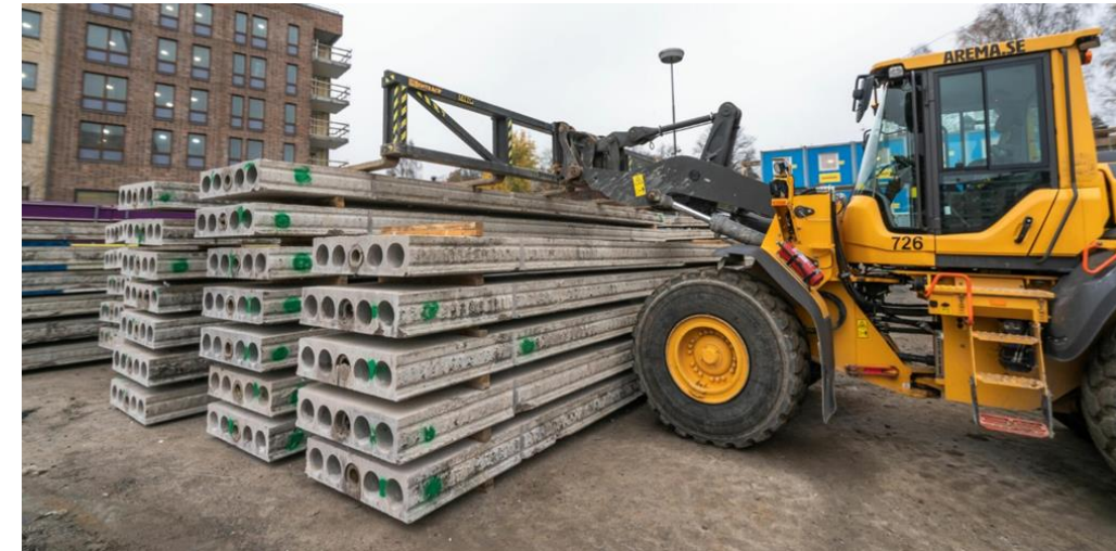
Stacked reclaimed precast concrete planks from a pilot project as part of the Aterhus project based in Sweden
