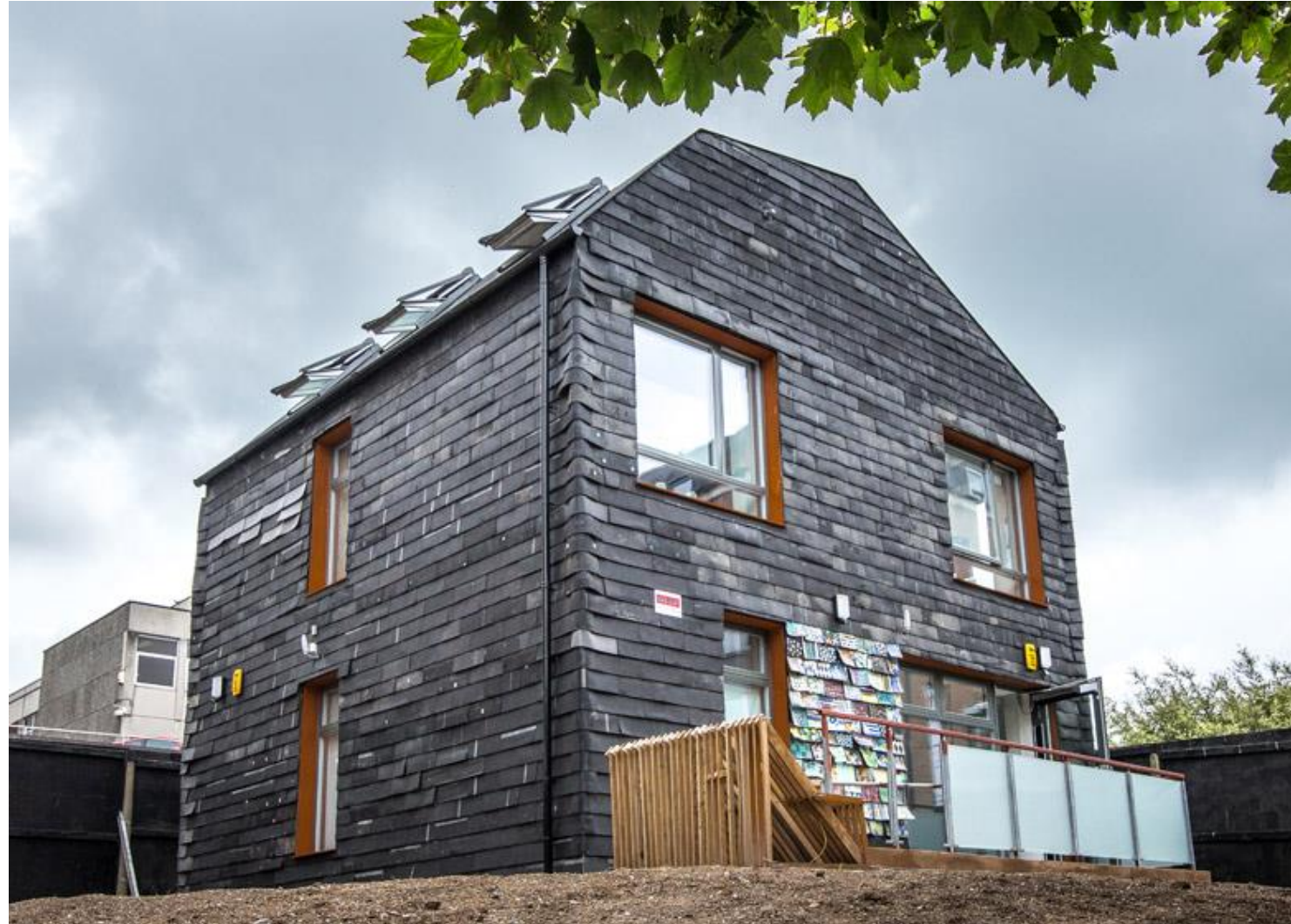
Brighton Waste House – timber reused for structural frame. House constructed from over 85% waste material.
